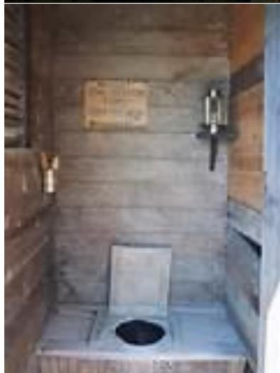
An outhouse operates differently from a septic tank in that the pit is not normally filled with standing water. The solids act as a sponge to retain moisture but also are exposed to open air, allowing for insects and earthworms to feed on the wastes which would not be possible within a septic tank. Septic tanks also tend to contain only organisms that can survive anaerobic conditions, while the open outhouse pit can sustain both aerobic and
